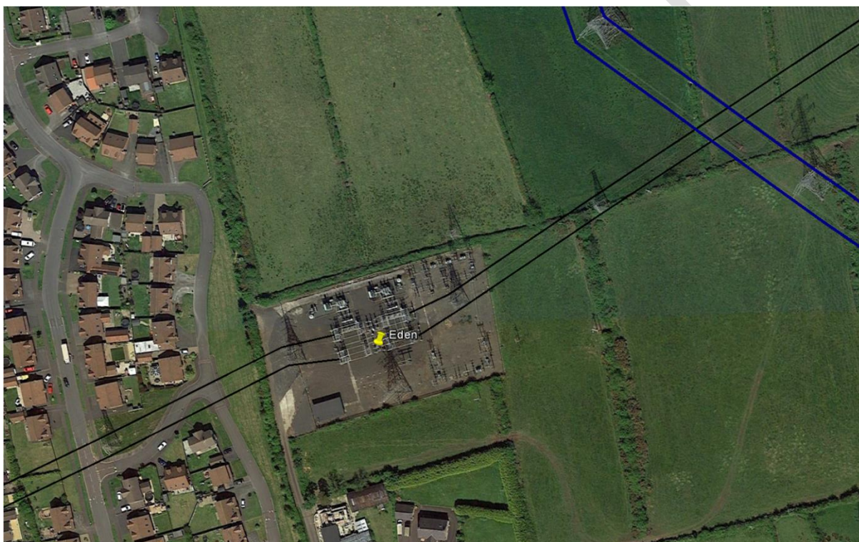
Figure 2.7: Eden 110/33 kV substation
