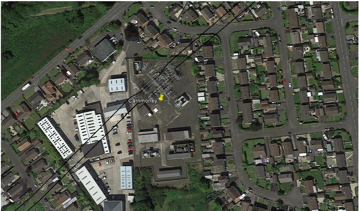
Figure 2.6: Carnmoney 110/33 kV substation
