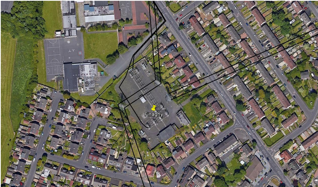
Figure 2.5: Finaghy 110/33 kV substation
