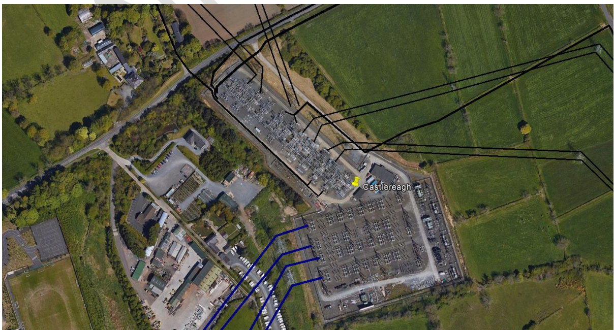
Figure 2.4: Castlereagh 275/110 kV GSP
